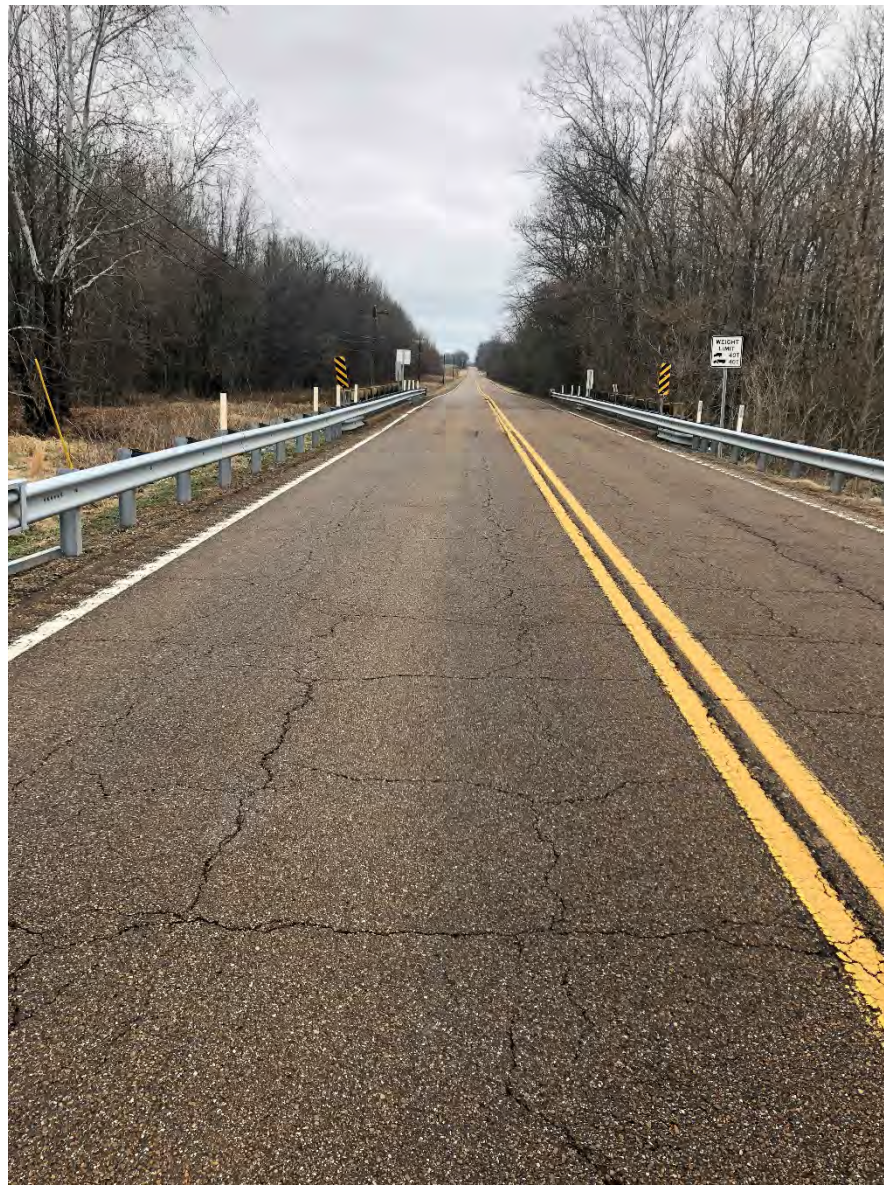
Eastbound Approach of Bridge
