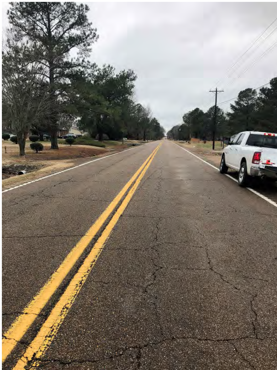
Looking Westbound from Bridge
