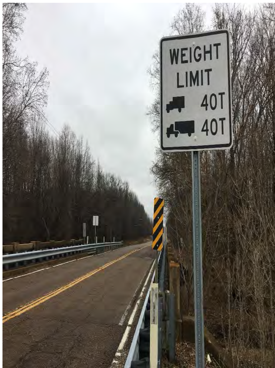
Weight Limit Sign at West Approach
