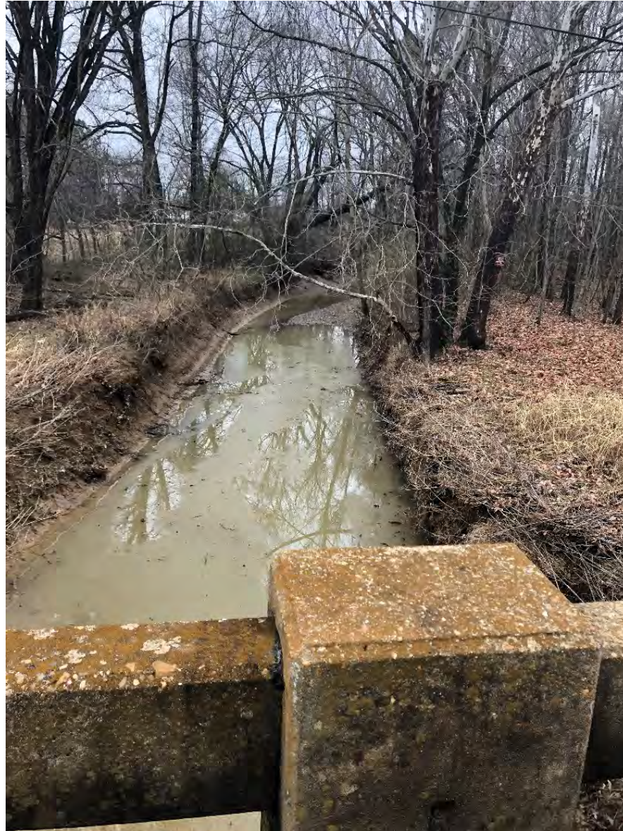
Downstream From Bridge
