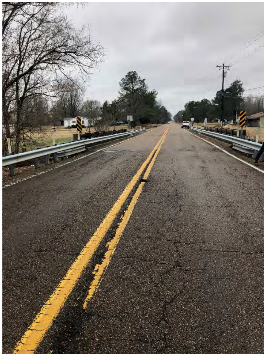
Westbound Approach of Bridge
