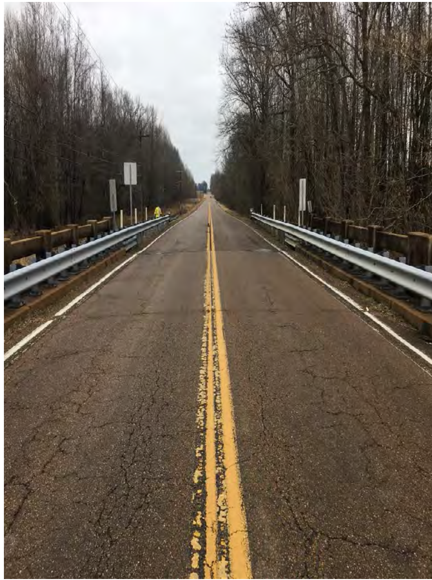
Looking Eastbound from Bridge
